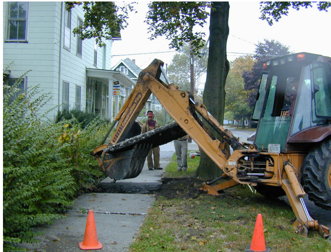
Fig. 1.20 Break-out zone with CU-Structural Soil™ under a sidewalk between a narrow tree lawn and adjacent landscape area
