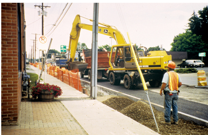
Fig.1.9 Installing CU-Structural Soil™ in Ithaca, NY in 1997
