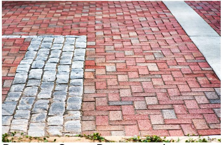
RUMBLE STRIP PAVERS IN LIEU OF THERMOPLASTIC PAINT WHERE NEEDED IN PAVER DESIGNED DRIVE LANES, THERMOPLASTIC PAINT IS SUBSTITUTED FOR A HIGH CONTRAST RUMBLE PAVER SUCH AS AN "OLD WORLD PAVER" STOP BAR PICTURED ABOVE, LOCATED ON Jefferson St.
