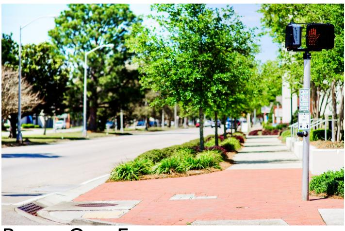
"BUMPED OUT" INTO THE ROADWAY TO ALLOW PLACEMENT OF STREET TREES WHILE REDUCING PEDESTRIAN EXPOSURE AND INCREASING TREE CANOPY COVERAGE ALONG PALAFOX
