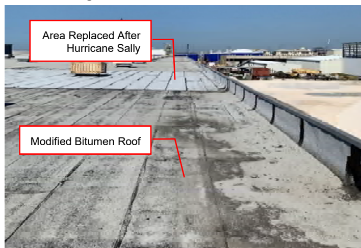
Figure 7: Roof Deck Warehouse #8
