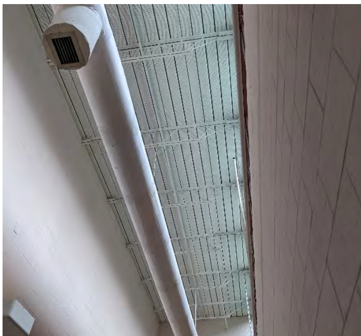
Figure 16: Roof Framing - Bar Joists - Vickrey Center Offices
