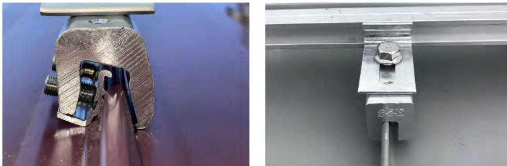
Figure 23: Standing Seam Metal Roof Clamp Mounts
