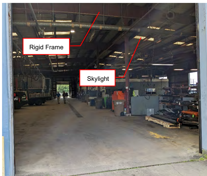
Figure 11: Roof Framing - Fleet Garage
