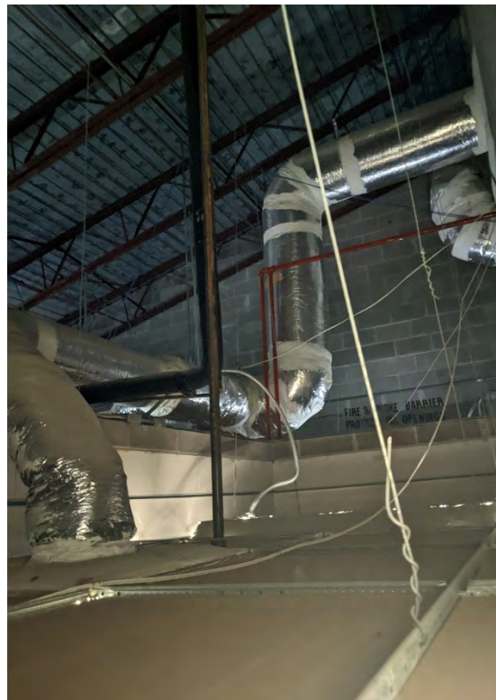
Figure 18: Roof Framing - Open Web Steel Bar Joists - Vickrey Center
