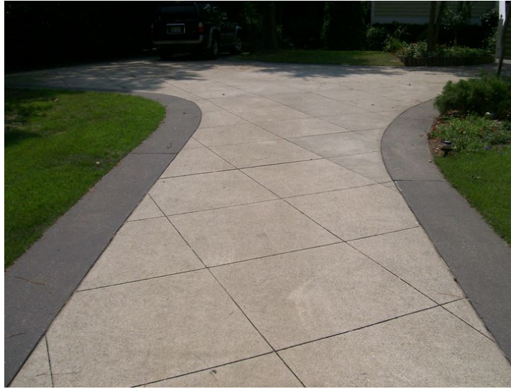
Unique angled concrete scoring patterns
