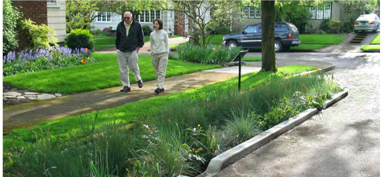
Curb extension with bioswale example that retains existing drainage infrastructure
