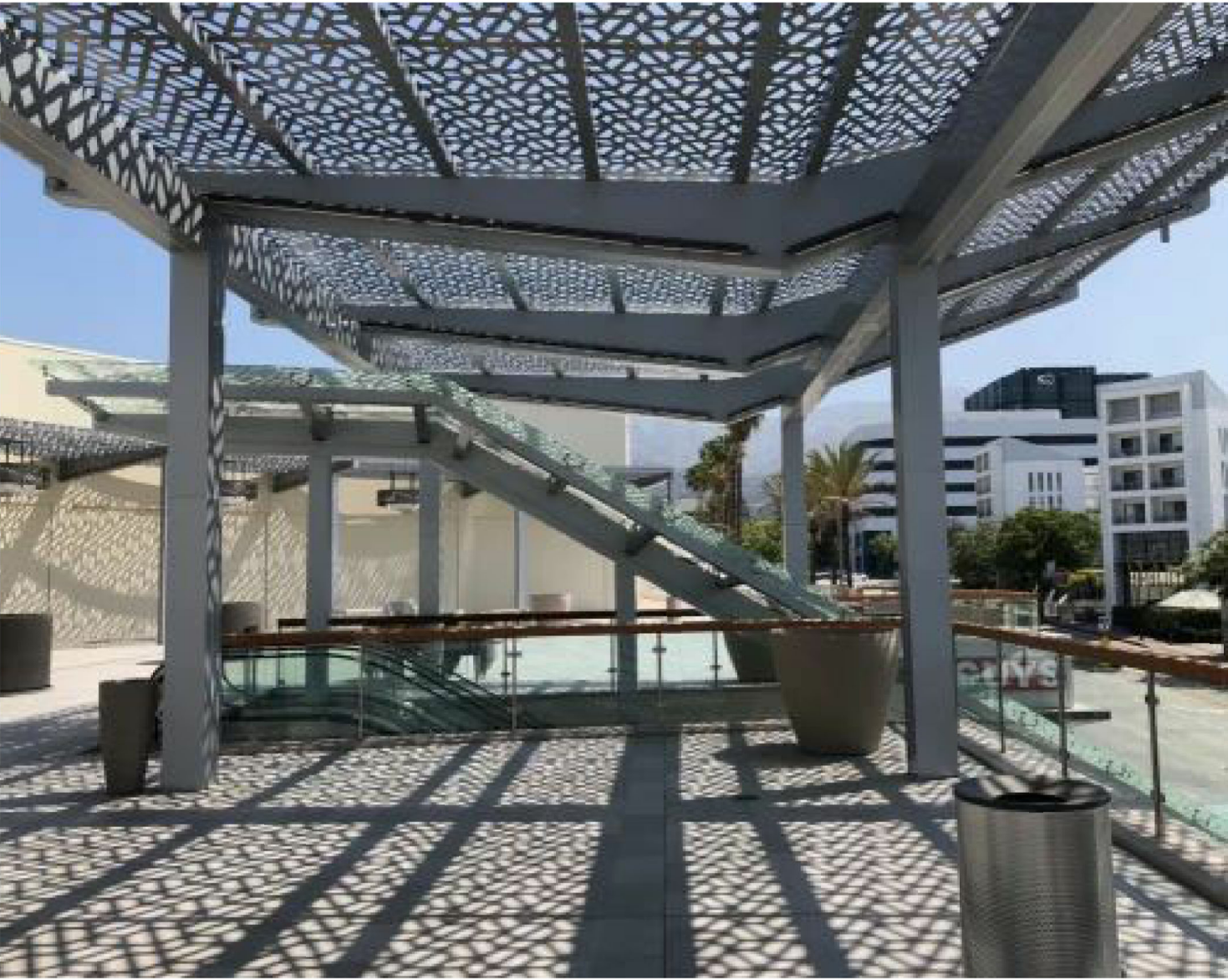
LASER-CUT METAL PANELS, PARASOLEIL OR SIMILAR POWDERCOATED, WEATHERED STEEL OR ALUMINUM TO COORDINATE WITH WAYFINDING DESIGN; STEEL POWDERCOATED POSTS
