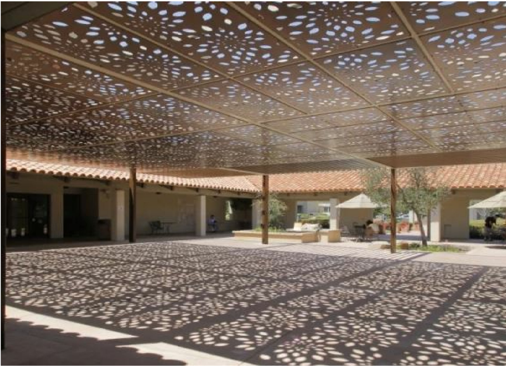
LASER-CUT METAL PANELS, PARASOLEIL OR SIMILAR POWDERCOATED, WEATHERED STEEL OR ALUMINUM TO COORDINATE WITH WAYFINDING DESIGN; STEEL POWDERCOATED POSTS
