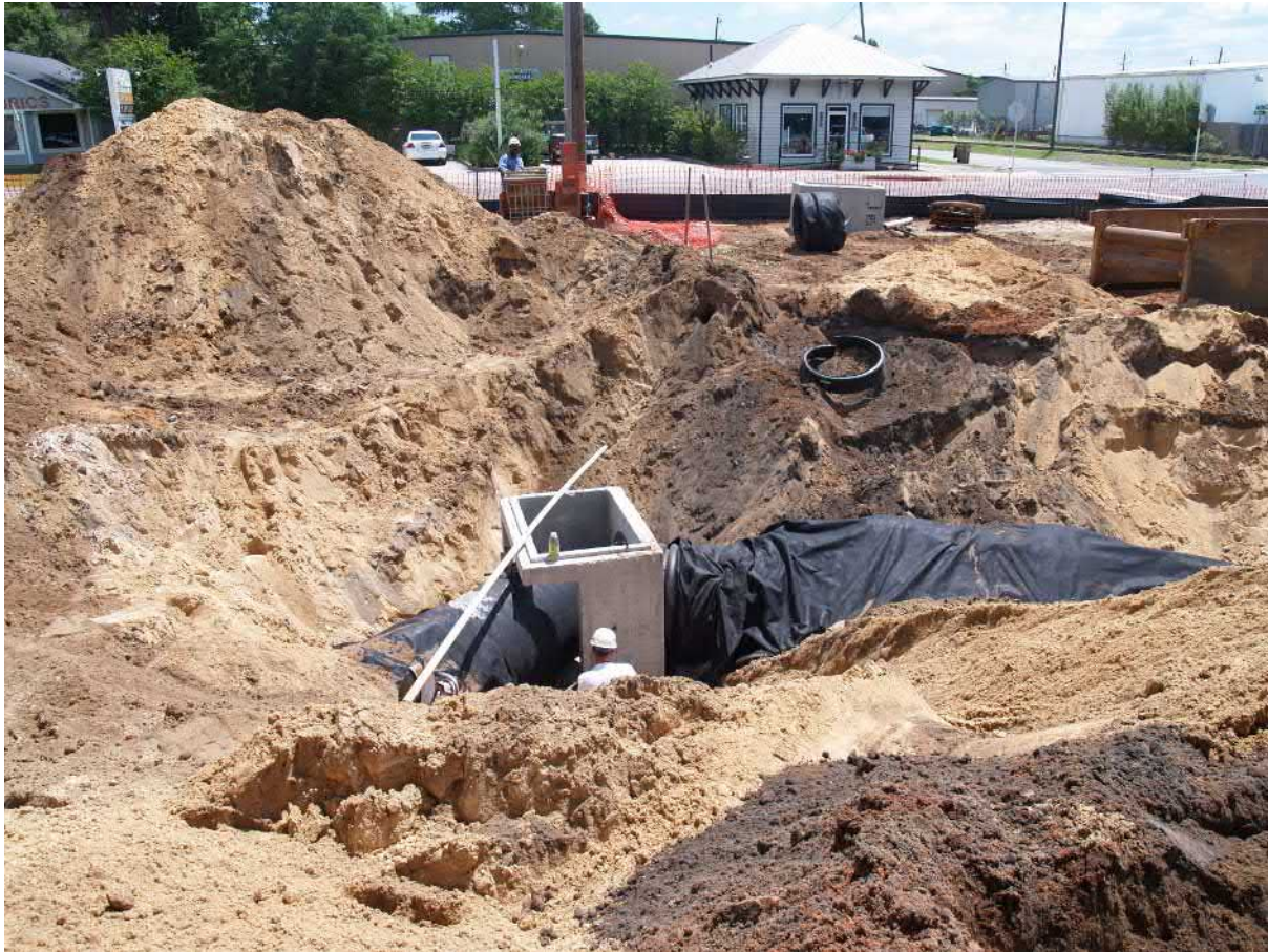
stormwater management is a criteria of the City - DUH appreciates sub-surface retention when needed
