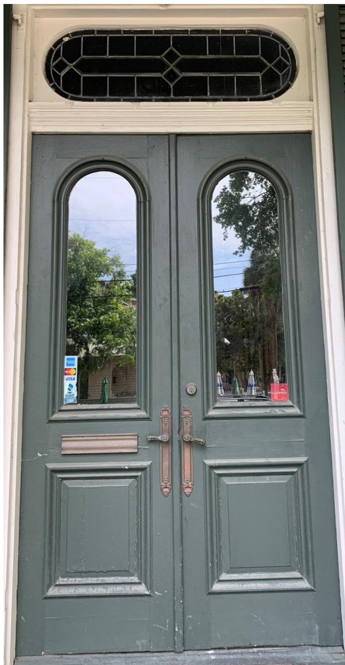
Front Doors to be refurbished or replicated with Impact Glass-color is Inkwel
