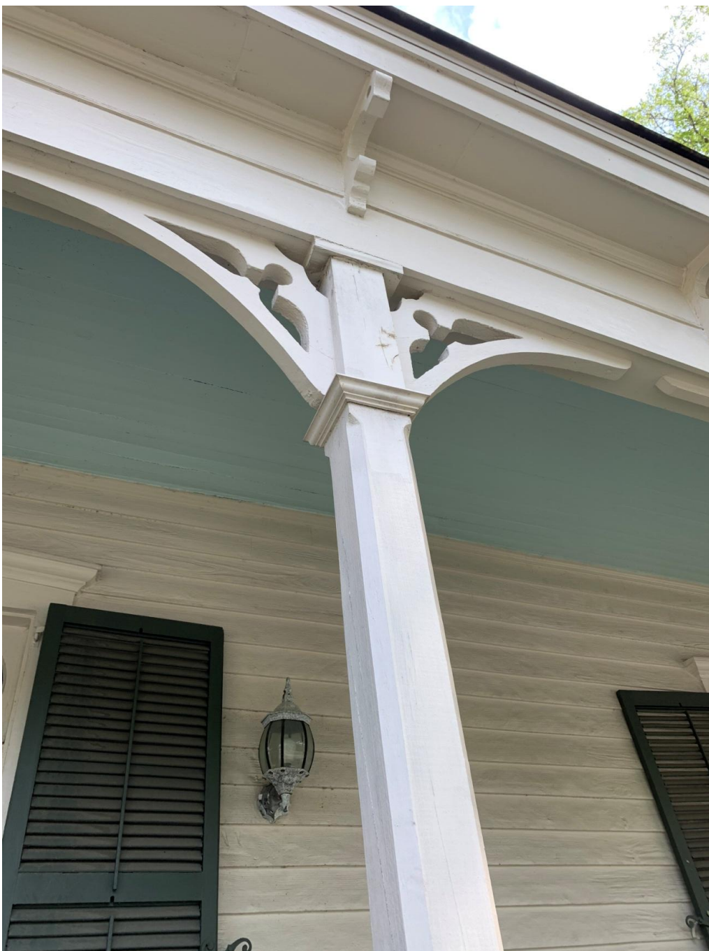
Porch Brackets and Column to be replicated and refurbished
