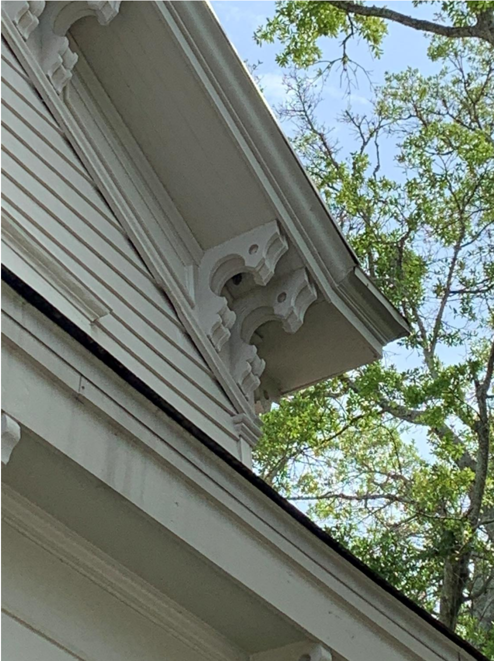
Corbels to remain and be refurbished or replicated
