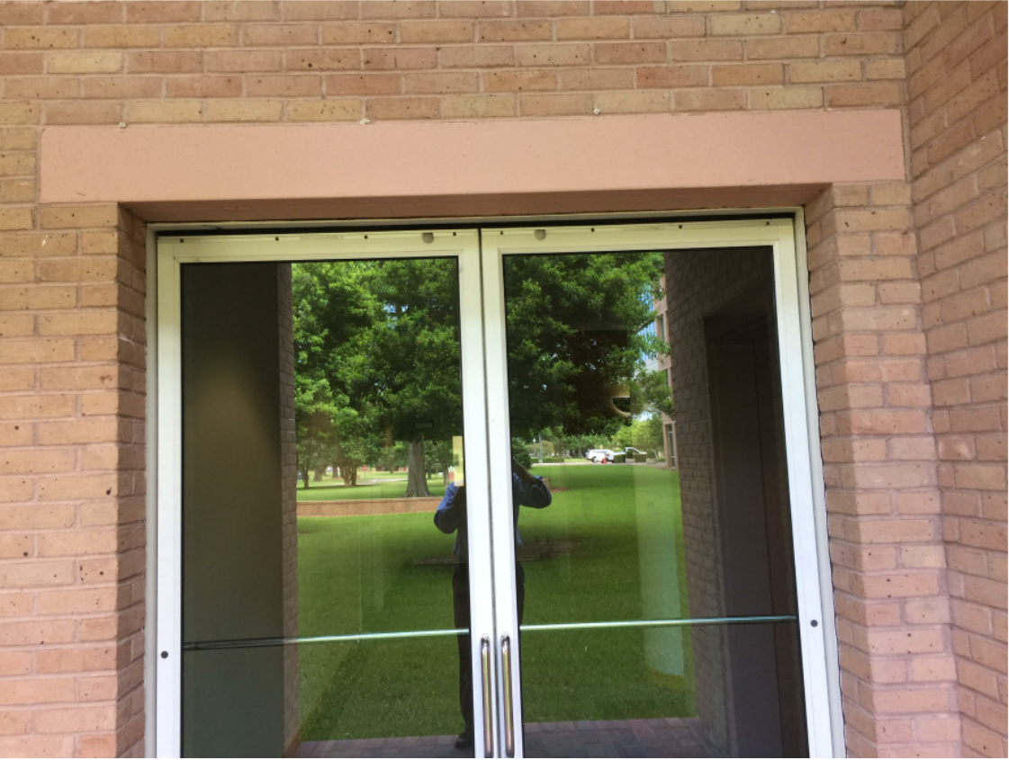
EXISTING BUILDING BRICK AND CONCRETE LINTEL
